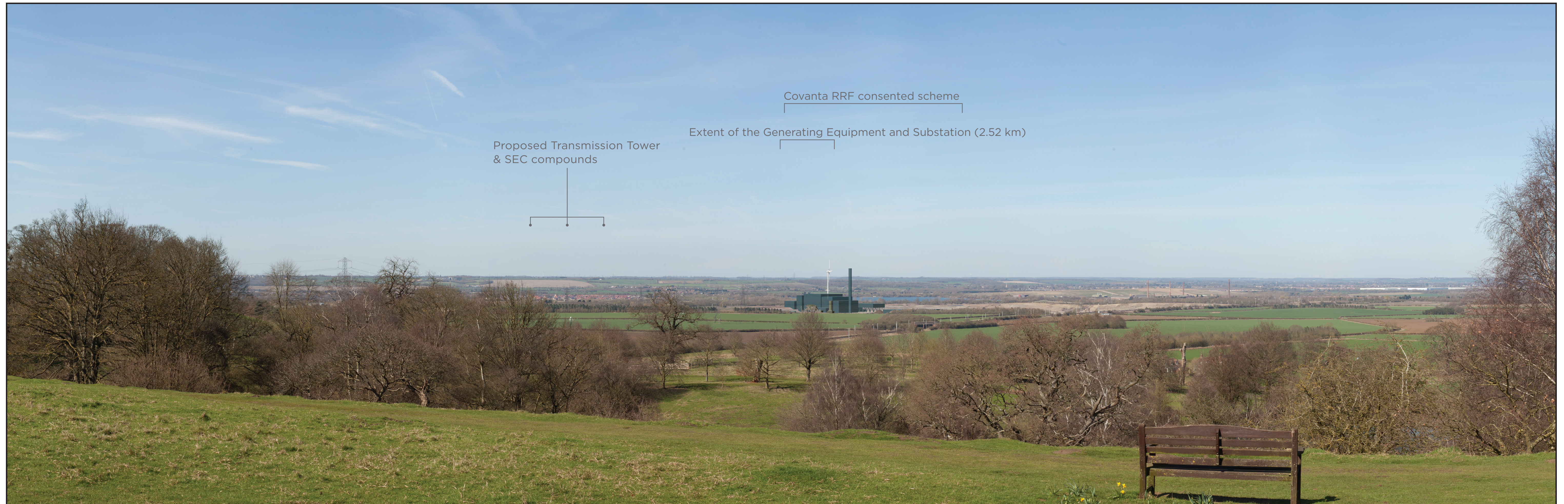
Photomontage view from Amphill Park, Katherine's Cross showing the Project and consented Covanta RRF scheme. (72 degrees horizontal field of view, 64 cm viewing distance). View direction 332 degrees. (Cylindrical projection).
